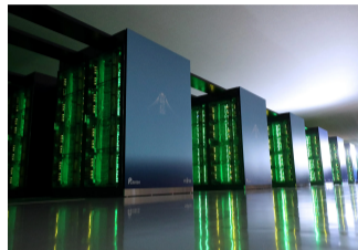
Japan's Fugaku supercomputer
